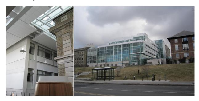
• The western side of the building is constructed with a double glass curtainwall system with integrated solar shading devices to control heat loss and gain.
