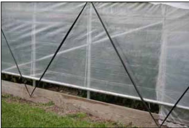
Figure 27. Open vertical side wall.
