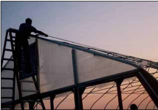
Figure 25a. Applying the plastic over the high tunnel superstructure.
