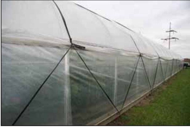
Figure 26b. Webbing applied over plastic to keep it from blowing in the wind.
