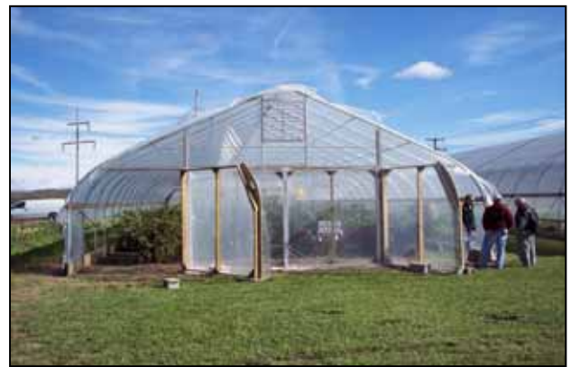
Figure 20. Hinged plastic covered tunnel doors.
