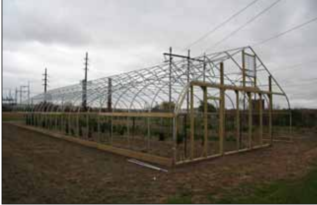
Figure 17. Peak-style high tunnel framing - side view showing batten boards.
