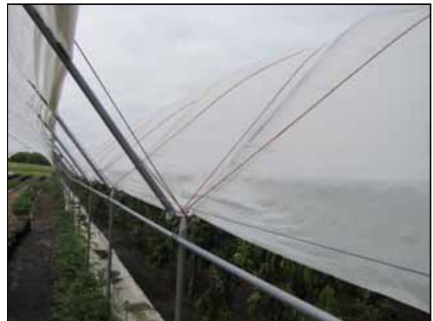
Figure 35. Multi-bay tunnels are vented by opening the ends and pushing the plastic up on the sides.
