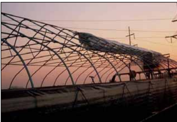
Figure 25b. Applying the plastic over the high tunnel superstructure.
