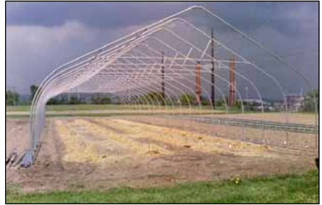
Figure 10. Peak-style high tunnel ribs (bows), Ithaca, NY.
