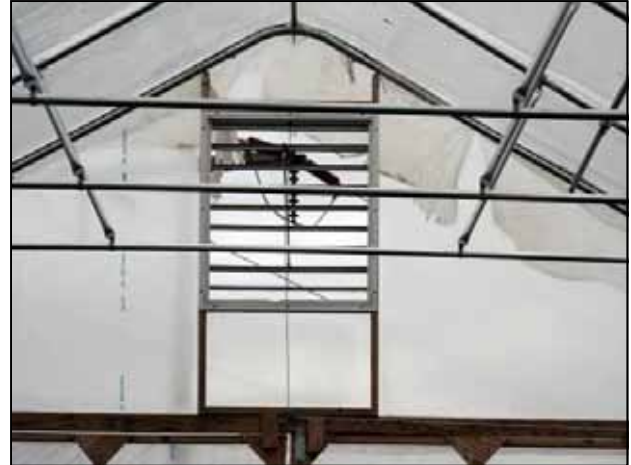
Figure 34. Venting the tunnel – peak vents.
