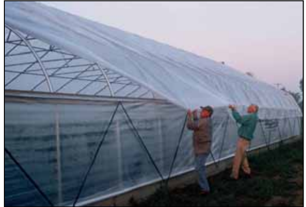
Figure 25c. Applying the plastic over the high tunnel superstructure.
