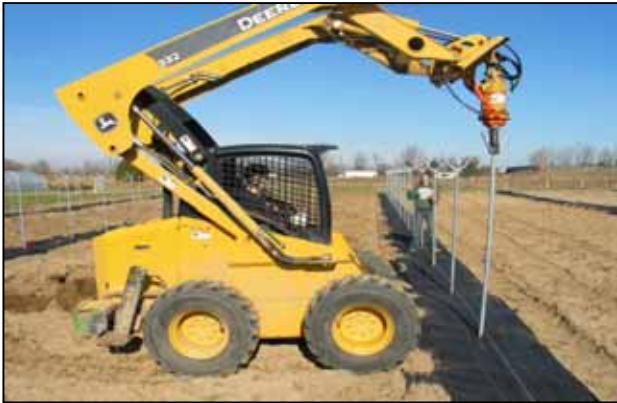
Figure 22. Multi-bay tunnels; leg posts are augered in at pre-marked positions.
