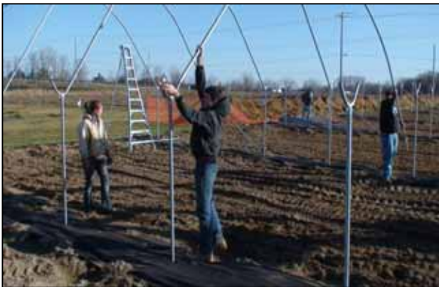
Figure 23. Multi-bay hoops are installed on leg posts.
