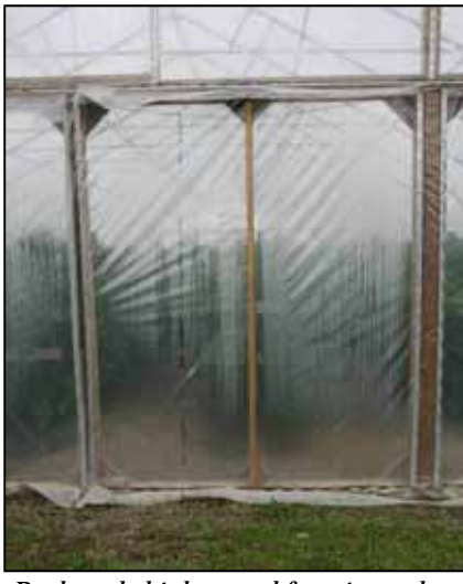
Figure 18. Peak-style high tunnel framing - close-up of end door.
