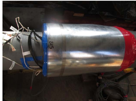
Figure 3.3. Pipe Joint with Protective Shielding
