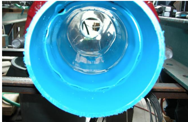
Figure 3.7. View of Interior of C2 Showing Pipe Spigot Pushing through Bell
