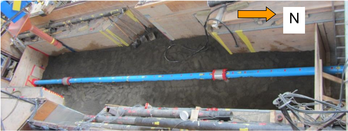
Figure B.1. Instrumented Pipe in Test Basin Prior to Backfill
