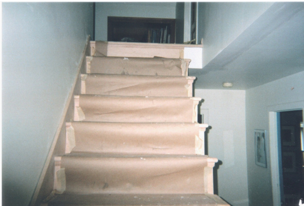
Figure 3. Purdy's picture of the stairs being built in his home.
