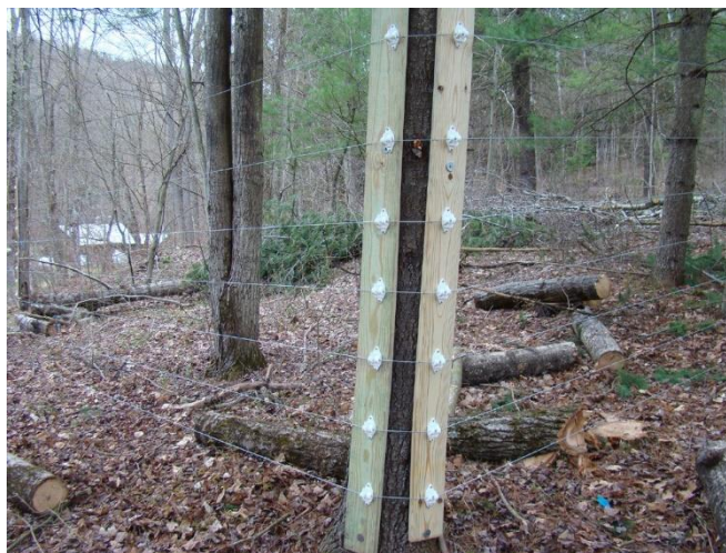
Figure 16. On abrupt corners, double batten boards may be necessary to protect the tree. Abrupt corners increase resistance when pulling wire around perimeter.
