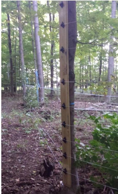
Figure 18. Use of a deck board as a batten strip and 8 strands of high-tensile wire
