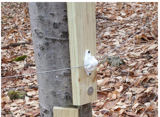
Figure 12. Batten strips can be custom fit as needed to tree shapes.
