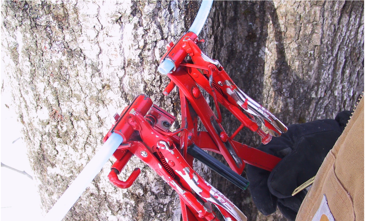
The double vice tool being used to insert the drop line T into the lateral line
