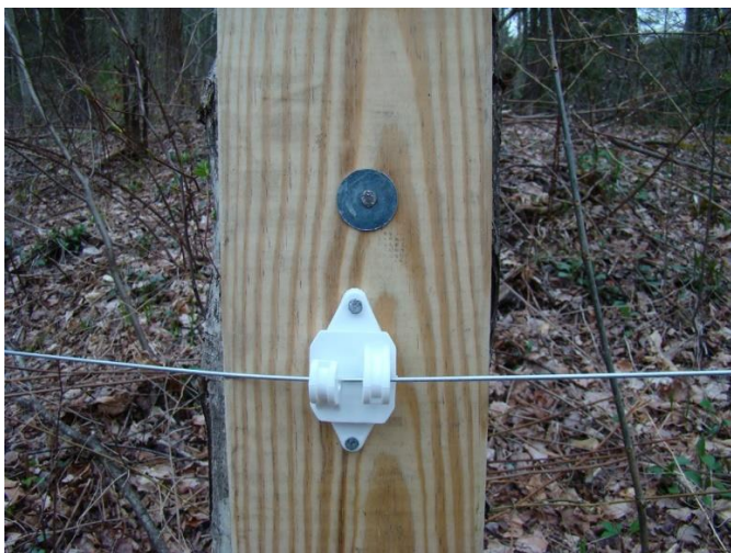
Figure 15. Pressure treated deck board (5/4 x 6) with fender washer, galvanized nail, and plastic clip for electric fence.
