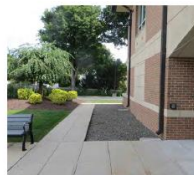
A two-foot wide vegetation free zone around buildings can reduce moisture problems. Photo: M. Frye
