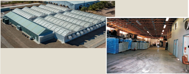
FIGURE 5. This headhouse includes material storage, restrooms, offices, a potting room, and an area to package plants for shipment.
