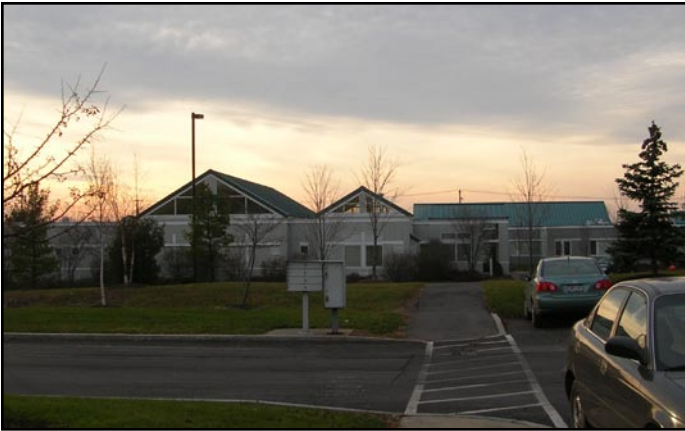
Figure 1.5. The facility has no signs or other forms of identification. There are still no signs when further proceeded.
