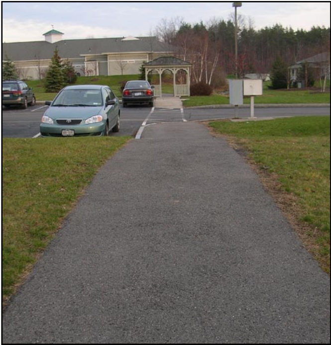
Figure 1.6. Unleveled paved path with no handrails.
