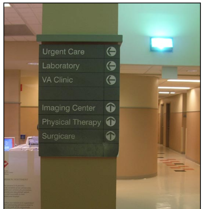
Figure 1.6. Main signage system at the East Campus. It lacks contrast, is too small, and has no brails.
